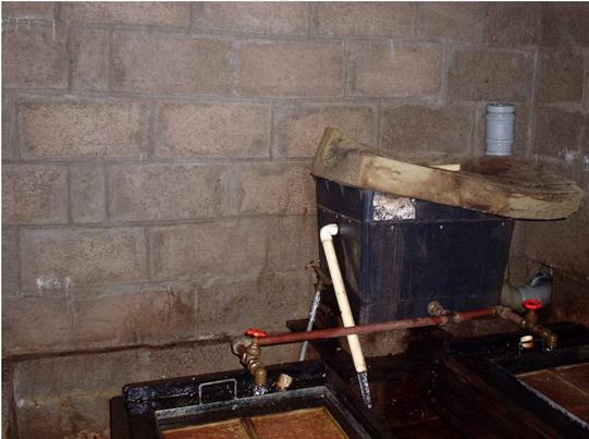
Water is also supplied to a 2 metre square Swedish tank and a 1.5 metre round tank which have been used for fry rearing. The wooden troughs contain 32 plastic trays with a capacity of 160,000 ova.
