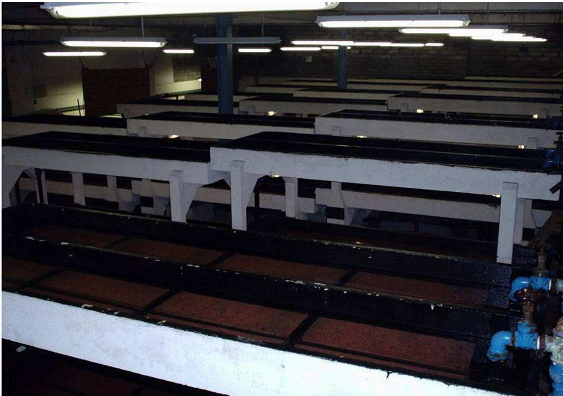
The Contin Hatchery contains 32 troughs each with three tiers and a separate water supply. There are also 8 2m tanks used for first feeding salmon fry. The total capacity of the Contin Hatchery is 4 million ova.
