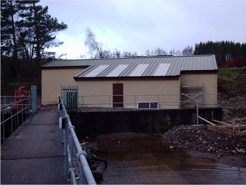
The broodstock unit is supplied with water by two submersible pumps from the Blackwater and contains 10 4m tanks with a capacity of 1,500 salmon.
