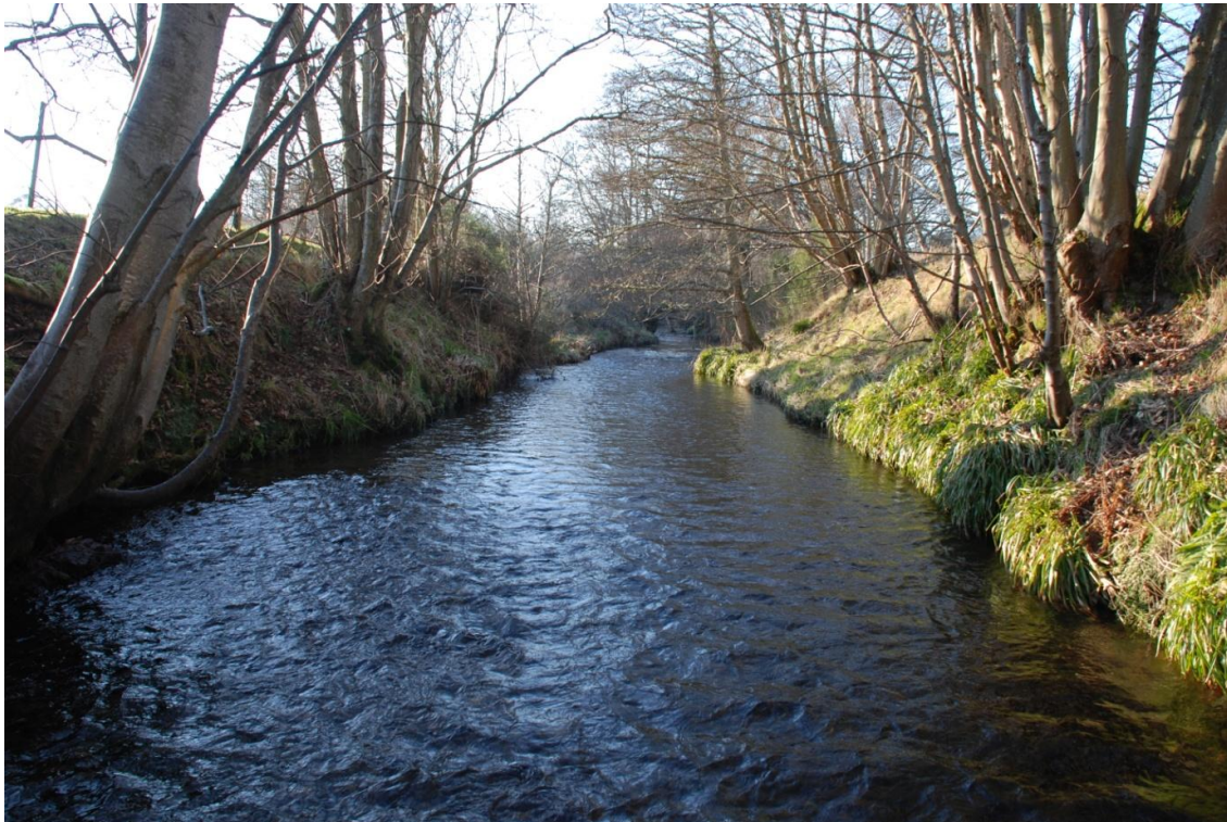
Picture 1, showing the section between Foderty House and Railway Bridge. Straight channel constrained within flood banks resulting in a uniform depth with limited in-stream habitat diversity and compacted bed.
