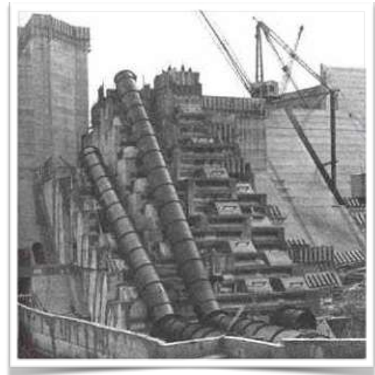
The four Boreland lifts being constructed at Orrin Dam
