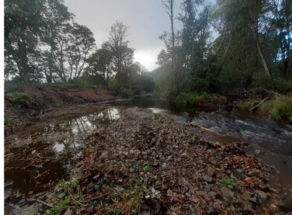
Balnagown obstruction removed.
