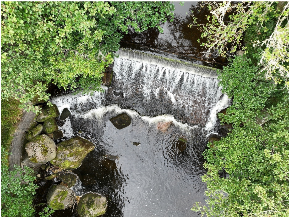
Figure 1: Marybank Weir on the Balnagowan, pre demolition, summer 2024.
